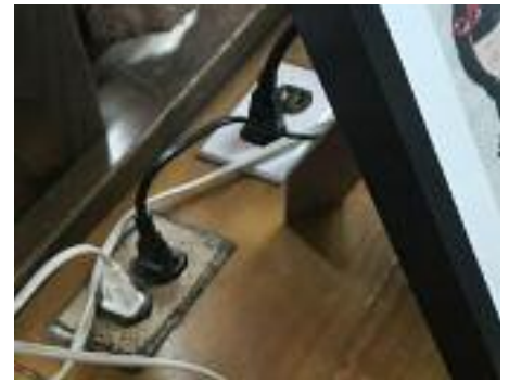
I also have outlets on built-in cabinets in my office. (Please ignore the outlet cover that has seen better days.)
